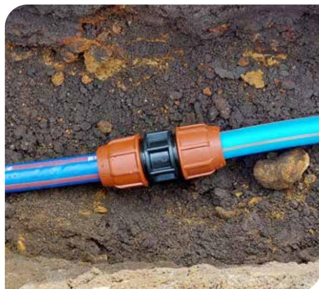
The PLASSON Barrier fitting has been specifically designed to accommodate all sizes between the tolerances stated in BS8588, the British Standard for water pipes in contaminated ground.
